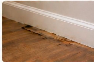
Floor damage from leaks
