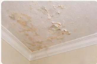
Ceiling bubbling & stains
